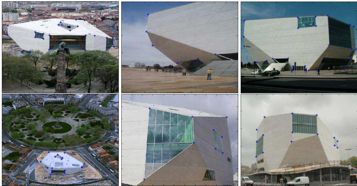
Figure 2.11: An image sequence of Casa da Musica in Oporto - a “piecewise planar” building. Blue dots represent feature location.
