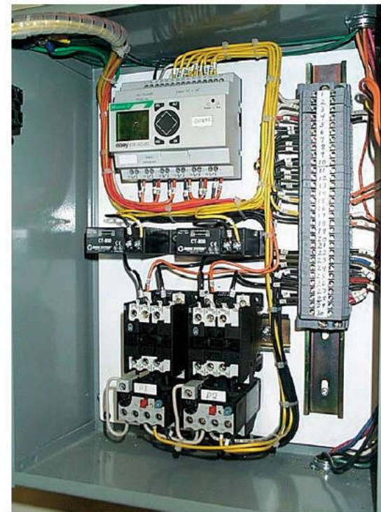
PLC control panel
