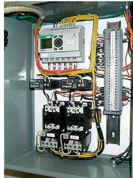
PLC control panel
