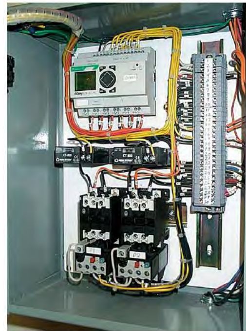
PLC control panel
